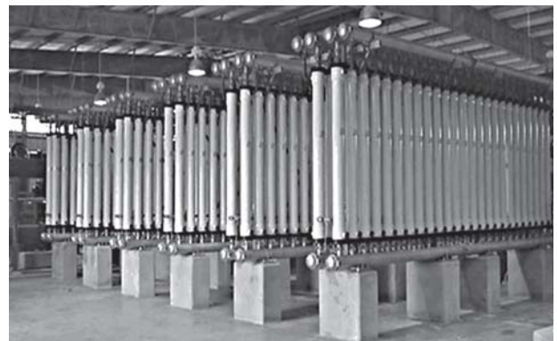
This is an example of a microfiltration plant similar to what will be built at the Mint Farm Industrial Park.
